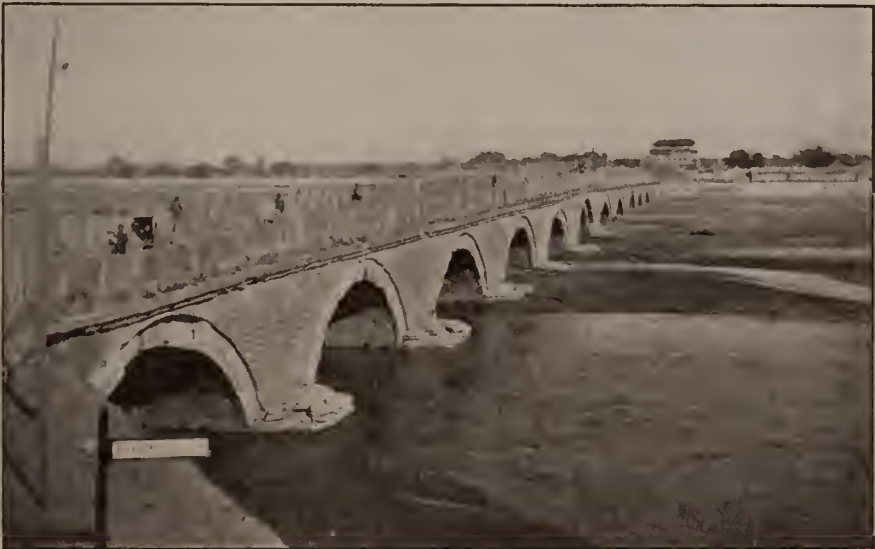
THE MARCO POLO BRIDGE AT LU KOU CHIOA
